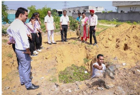
Dumping of Organic Waste
